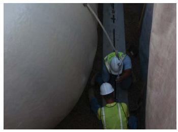
CSI deadmen include adjustable anchor points for easy positioning and installation.
