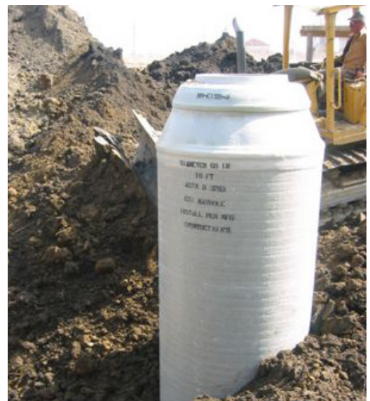
Fiberglass manholes are easier and safer because they are lightweight.
