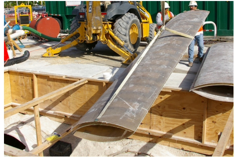
Panel sections are lowered into the existing tank.
