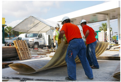
Prefabricated panels are prepared for tank entry.
