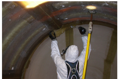
Joints are bonded together as the new inner tank is created, capable of being hydrostatically monitored.
