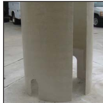
New inner wall includes doghouse cuts for existing piping
