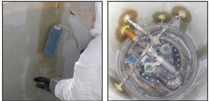
Layups applied to vertical seam and doghouse cutouts
