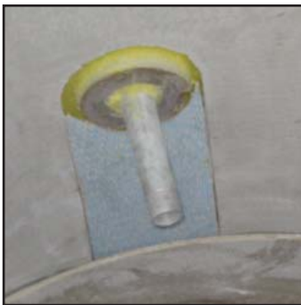
Separator material behind doghouse cut piping inserts
