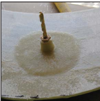
Drain fitting for annular space
