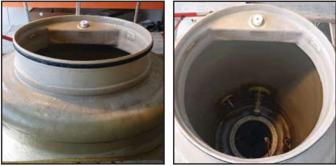
New double-wall sump top includes monitoring fluid reservoir
