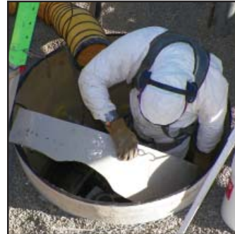
New collar inside sump
