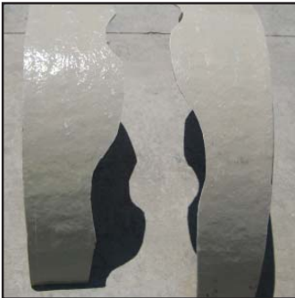
Collar cut to fit the curvature of the tank top
